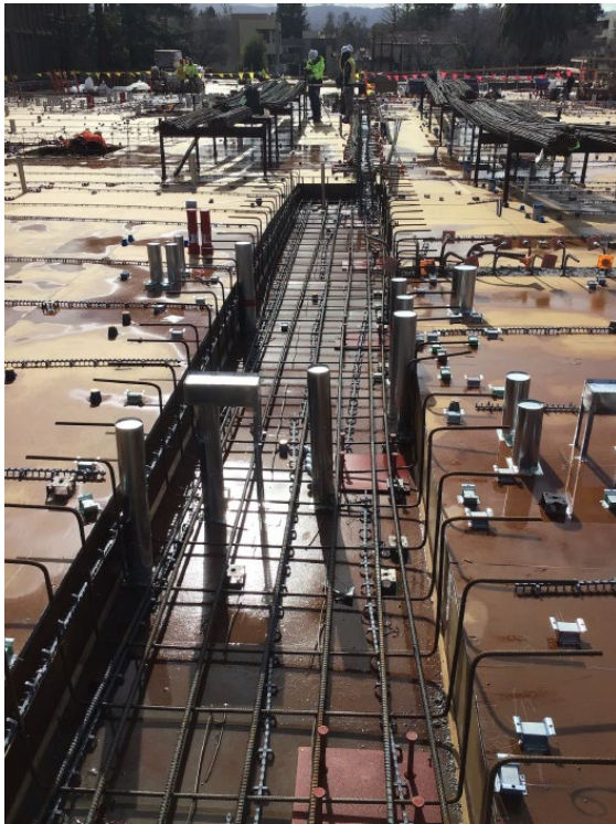
Figure 3 – Rebar installation at concrete podium
