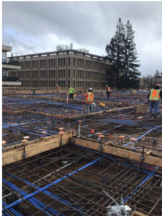
Figure 4 – Wide view of rebar installation at concrete podium
