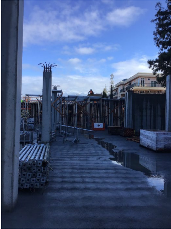
Figure 1 – Decking installation
