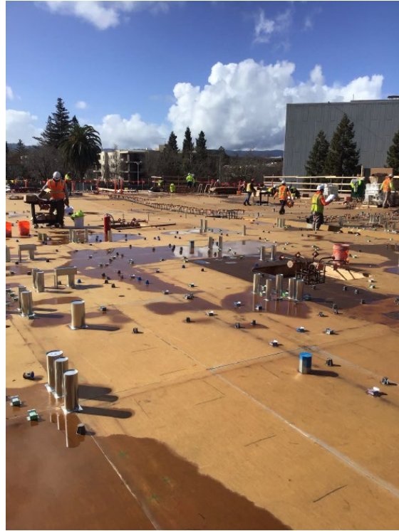
Figure 2 – Start of mechanical, electrical, and plumbing systems at concrete podium
