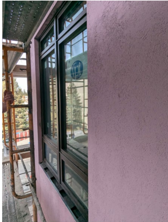
Figure 4 – Stucco Finish coat on Elevator Tower
