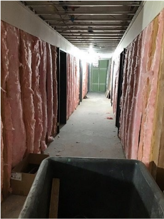
Figure 6 – Installed Corridor Insulation
