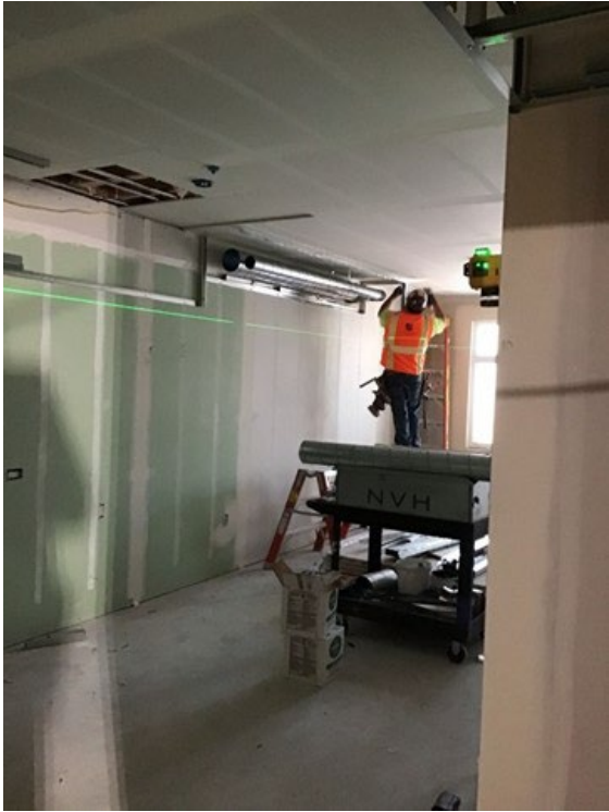
Figure 5 – Kitchen Soffit Framing
