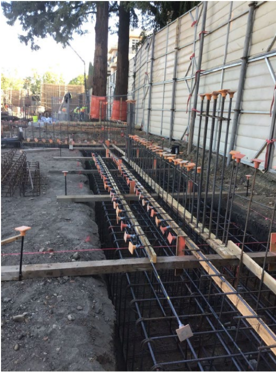
Figure 5 – Grade Beam Foundation
