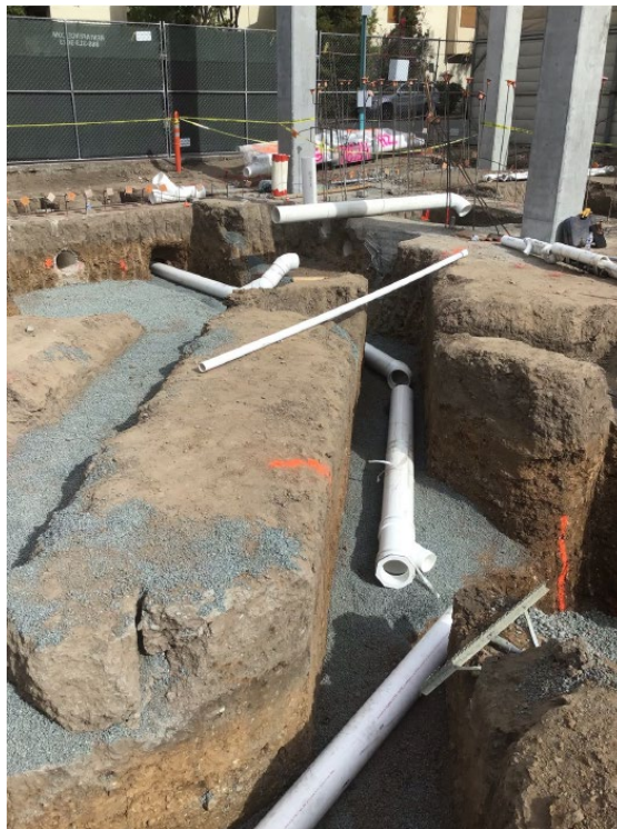
Figure 3 – Sub-Slab Utilities
