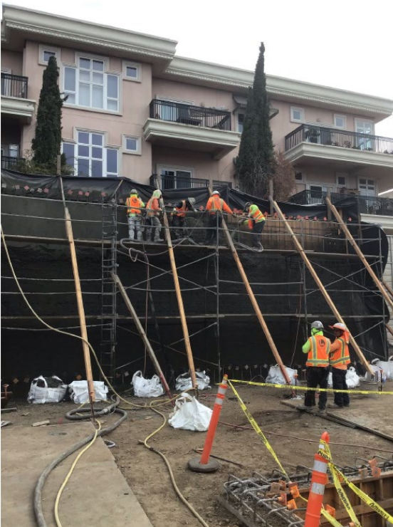
Figure 7 – Shotcrete Wall Placement
