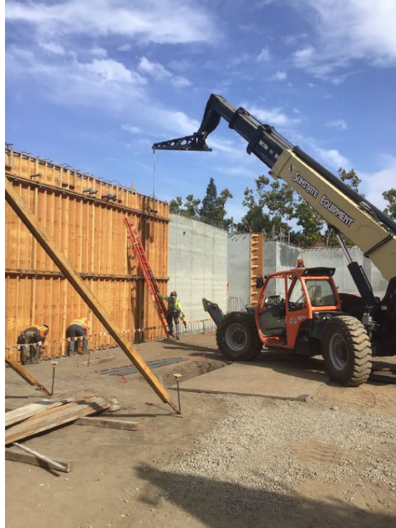
Figure 8 – Wall Panel Placement
