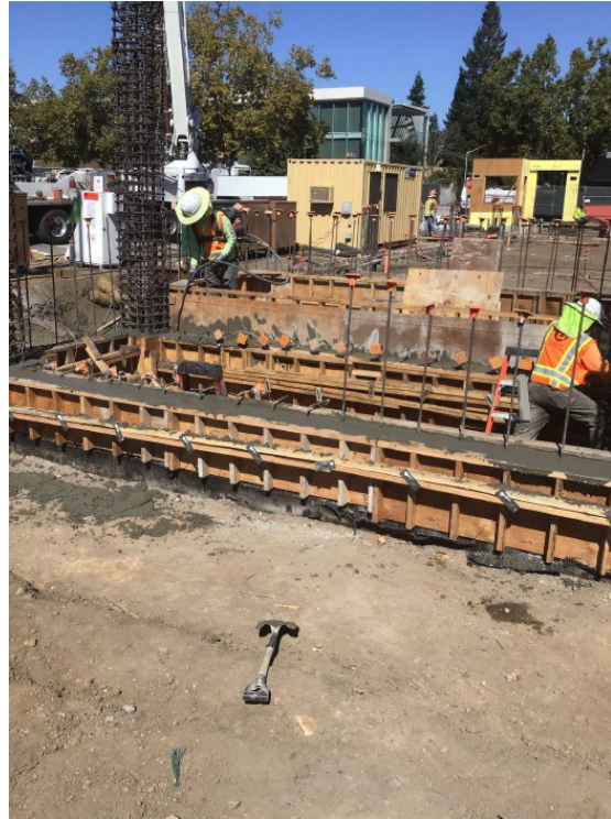
Figure 6 – Elevator Pit Rebar Columns
