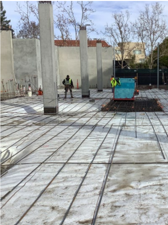
Figure 4 – Rebar installation
