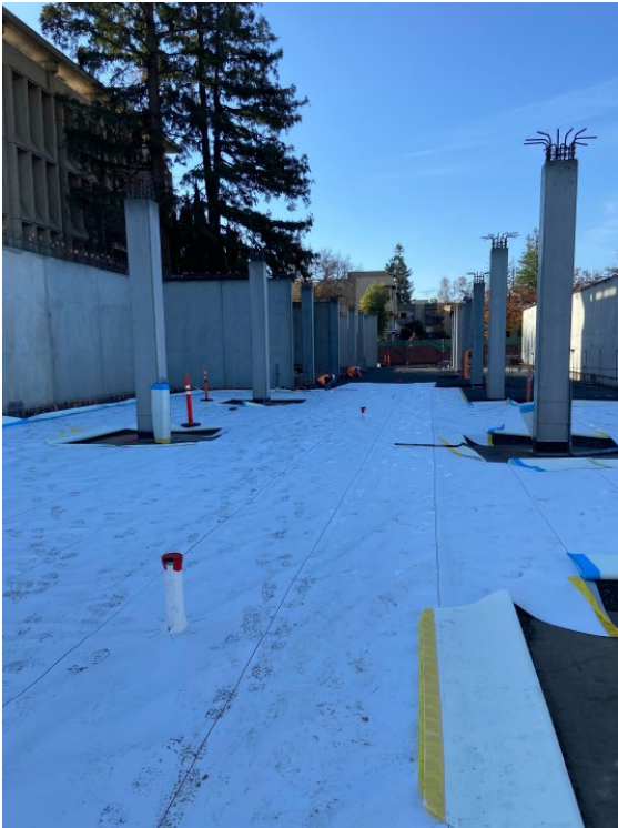
Figure 3 – Completed section of vapor barrier
