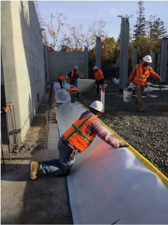
Figure 2 – Vapor barrier installation
