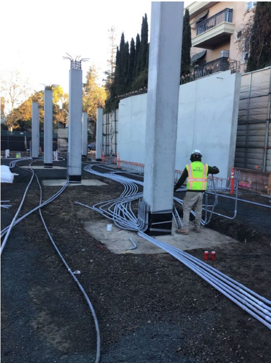
Figure 1 – Sub-slab utility installation
