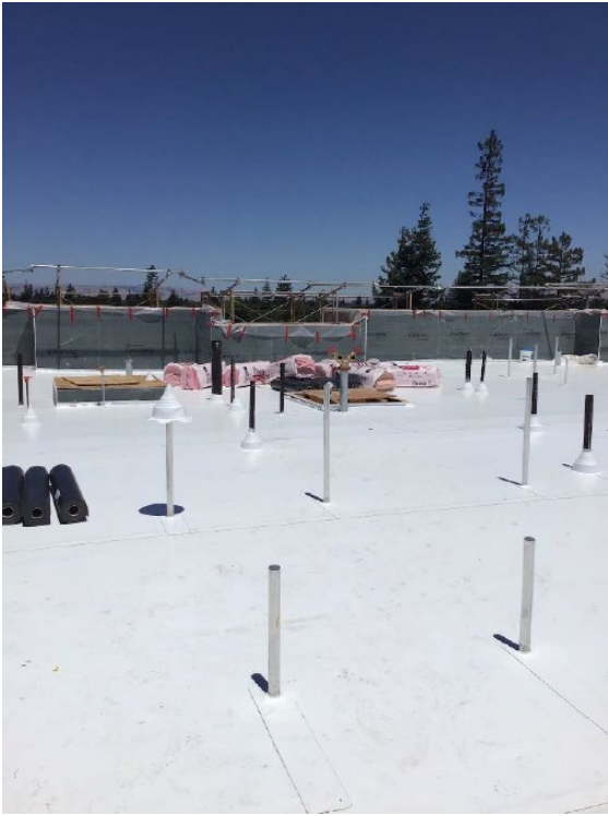
Figure 4 – Roof panel installation progress
