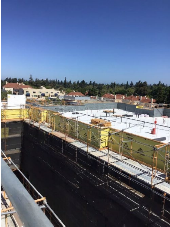
Figure 5 – Roof insulation progress
