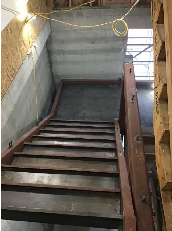
Figure 2 – Metal stairs at third floor
