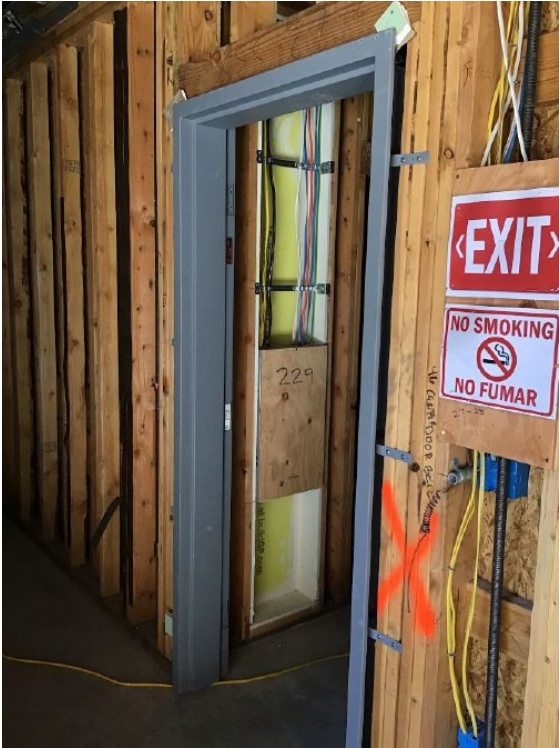
Figure 6 – Door frame installation
