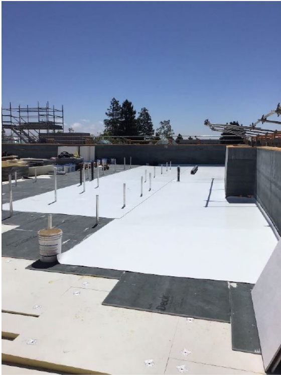
Figure 3 – Roof panel installation
