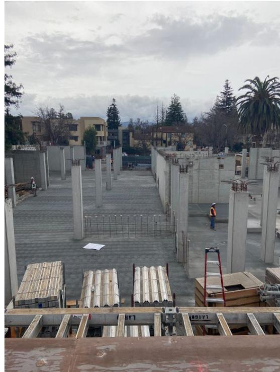
Figure 6 – Wide view of completed slab-on-grade
