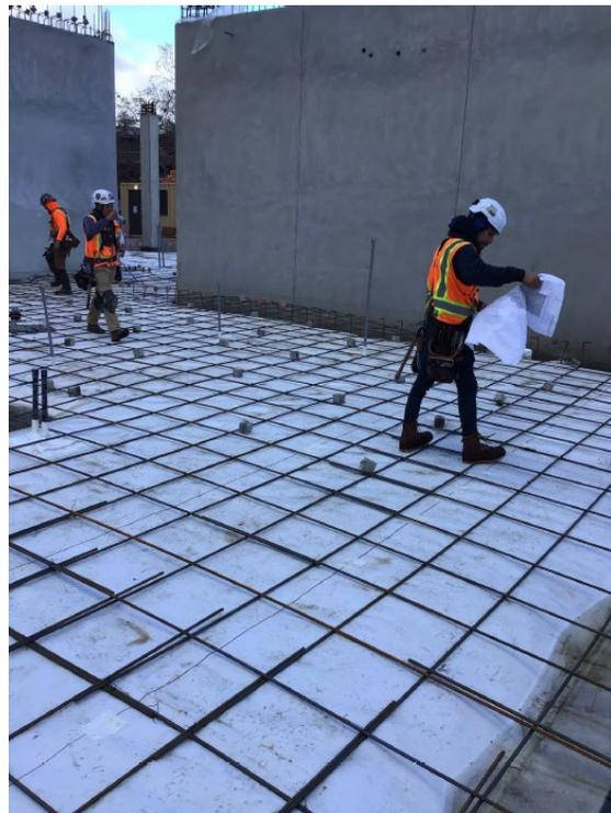
Figure 8 – Rebar structurally supporting slab-on-grade
