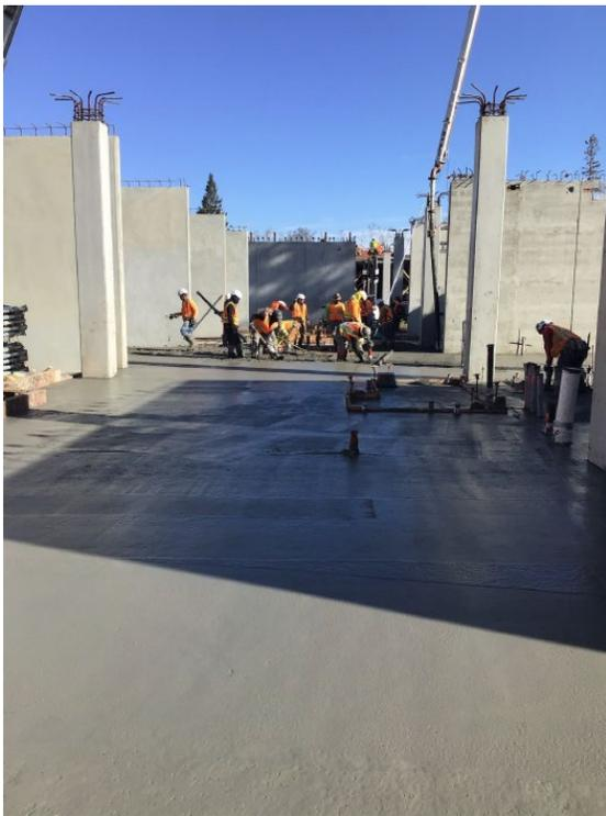
Figure 3 – Concrete pour for western slab-on-grade
