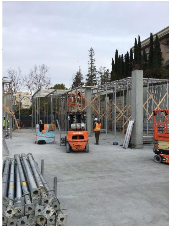
Figure 4 – Shoring over eastern slab-on-grade
