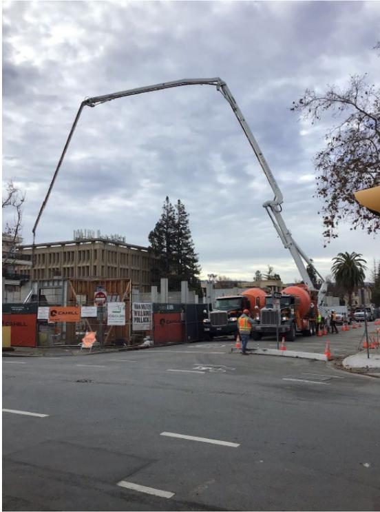
Figure 1 – Concrete pump
