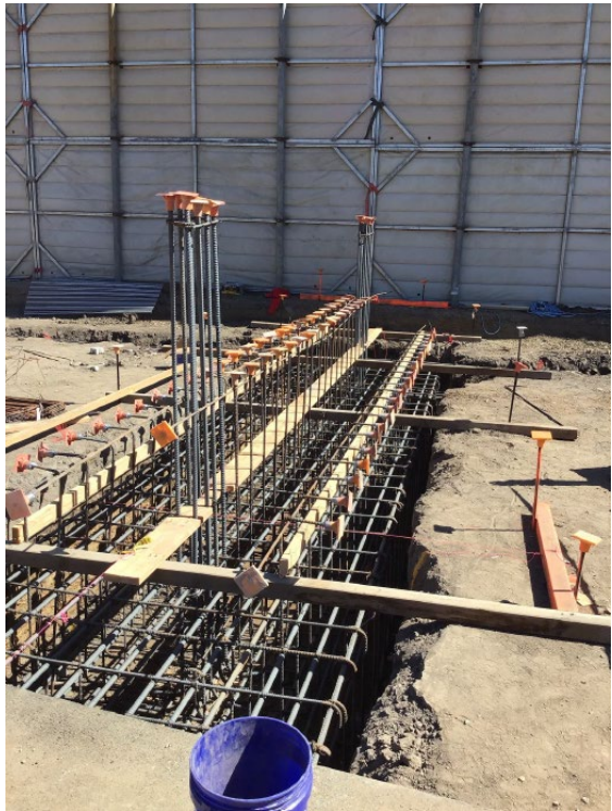
Figure 8 – Foundation Rebar
