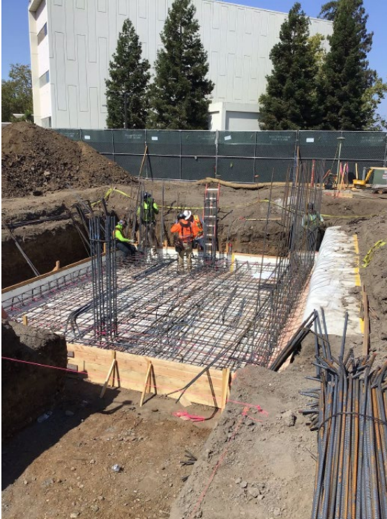
Figure 5 – Elevator Pit Rebar
