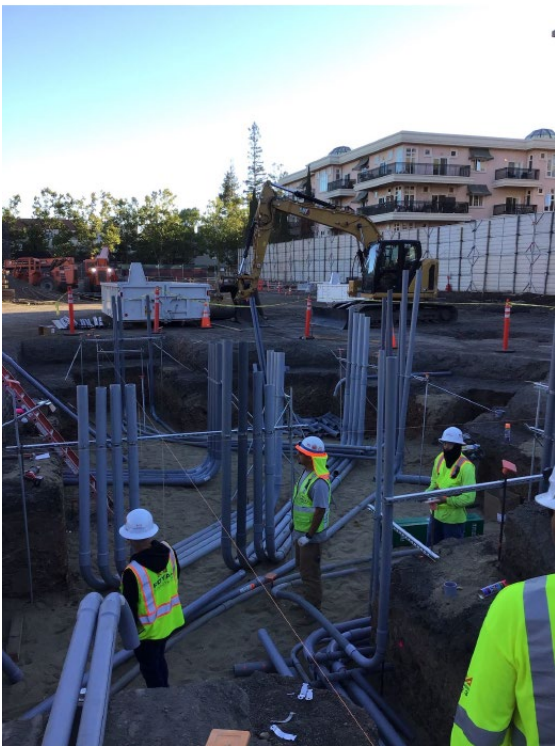
Figure 7 – Sub-Foundation Utilities
