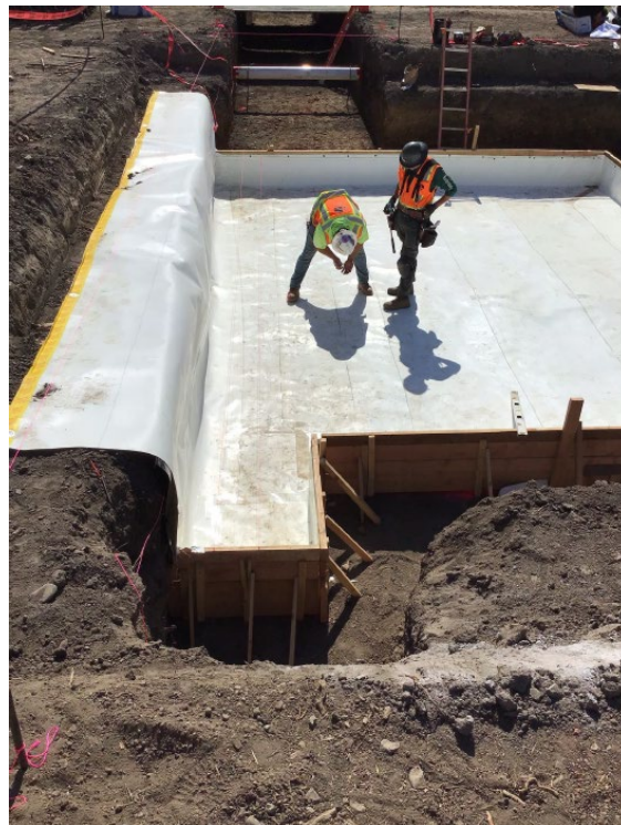
Figure 4 – Elevator Pit Waterproofing
