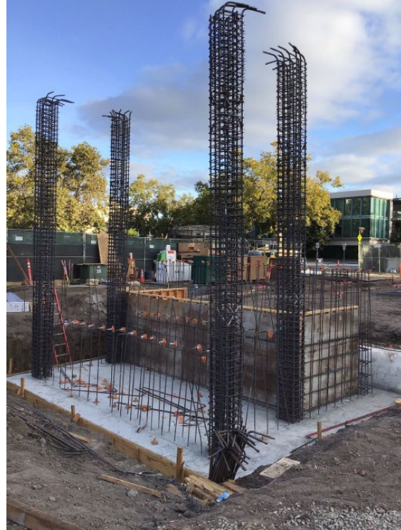
Figure 6 – Elevator Pit Rebar Columns
