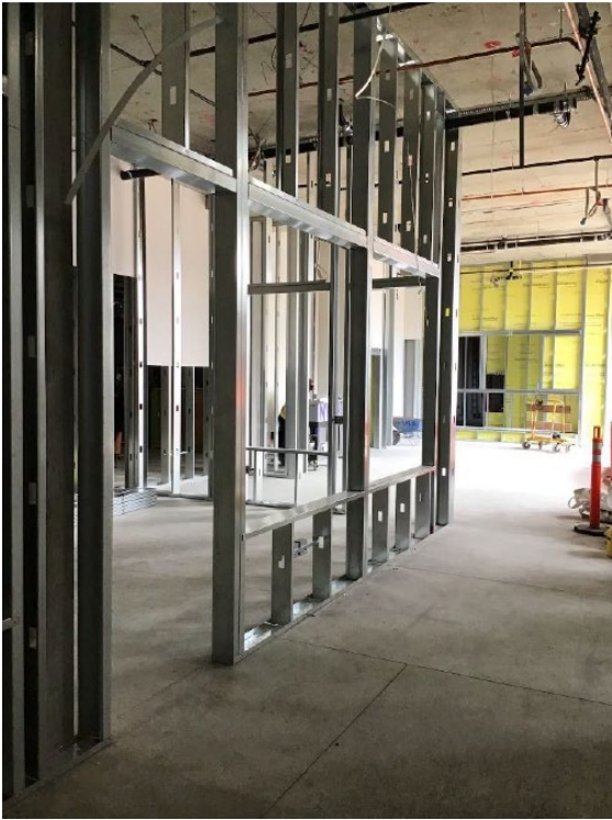
Figure 3 – Interior metal framing
