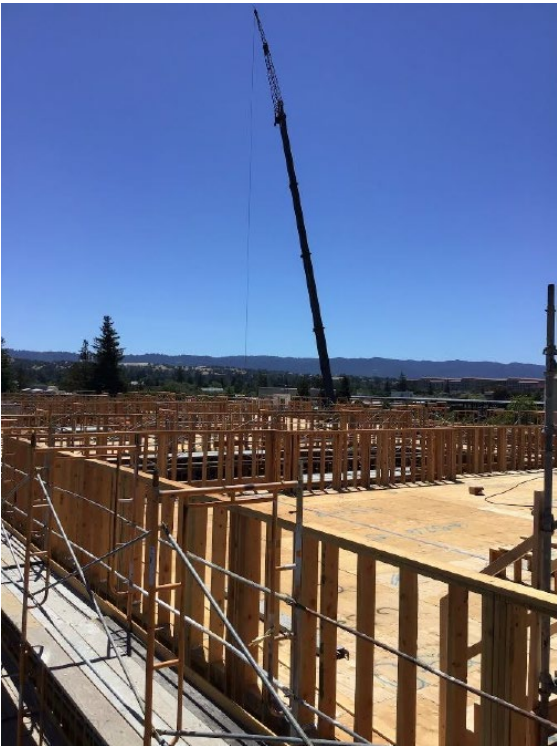
Figure 2 – Roof wood framing
