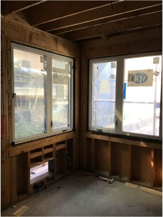
Figure 7 – Unit window installation
