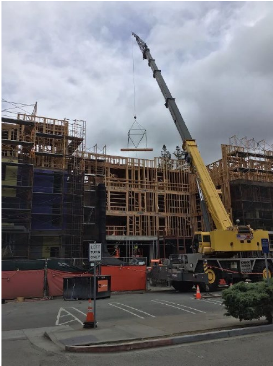
Figure 1 – Vertical wood framing
