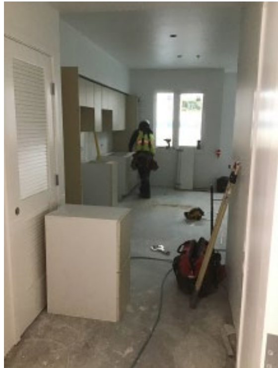
Figure 4 – Second floor kitchen cabinet install
