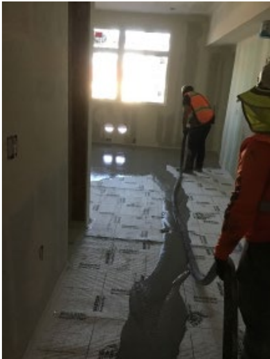
Figure 3 – Floor three gypcrete (subflooring)
