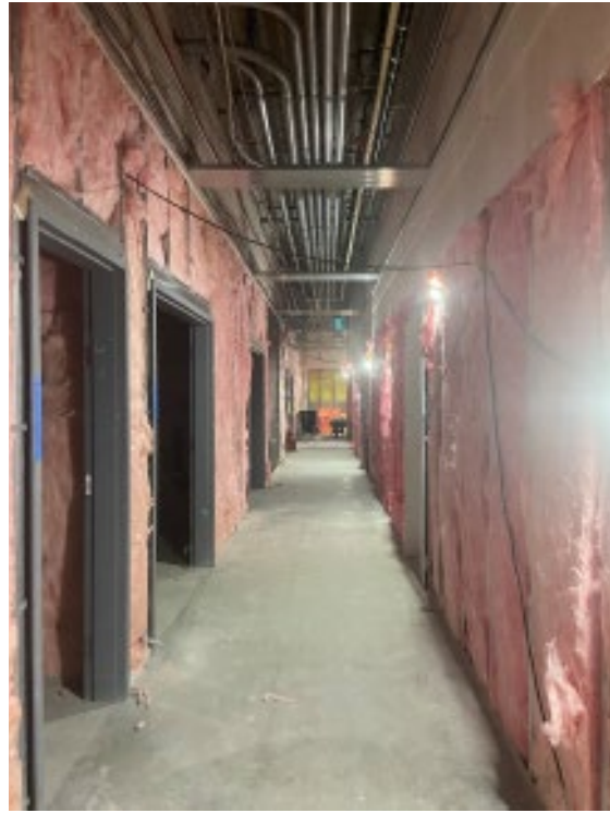
Figure 6 – continued insulation install
