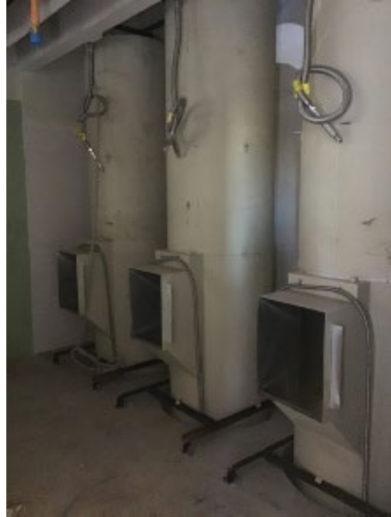
Figure 2 –Upper floor trash Chutes
