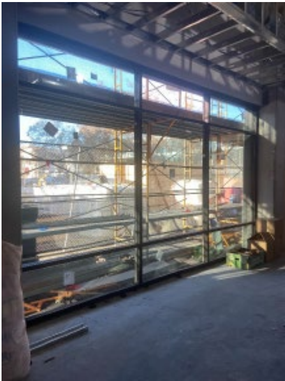
Figure 7 – Storefront window frame and glass installed
