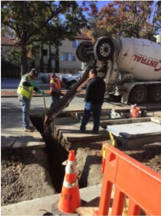
Figure 5 – Birch street utility work
