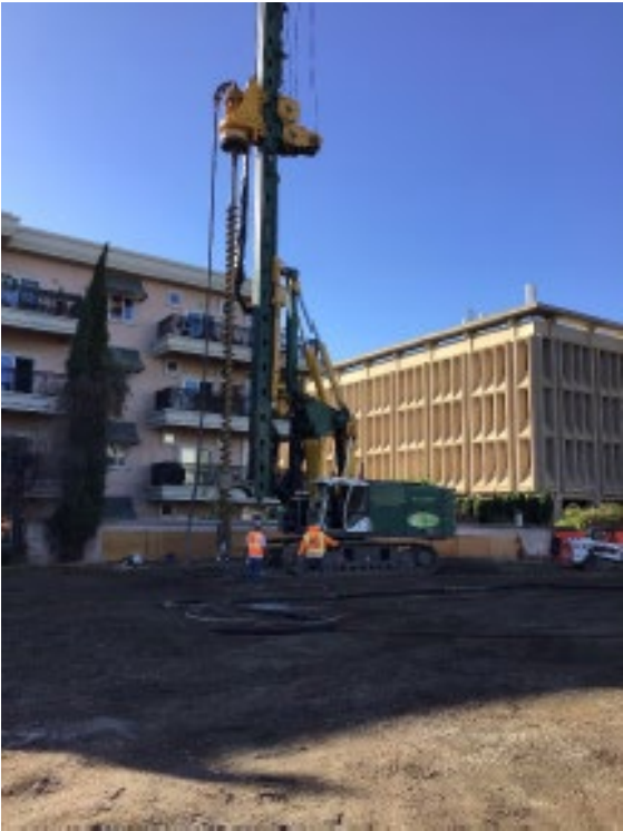
Figure 6 – Pier Drilling
